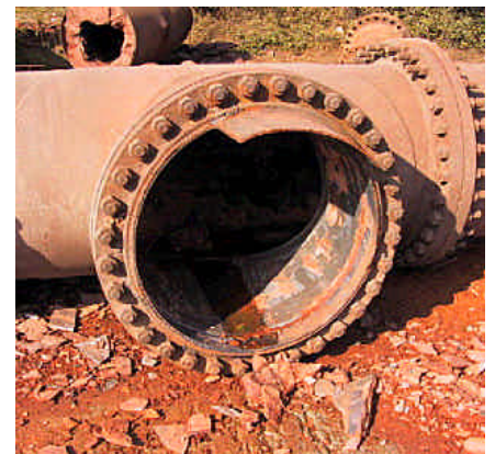
Heavily contaminated pipes blasted to smooth finish by tank cleaning head.
