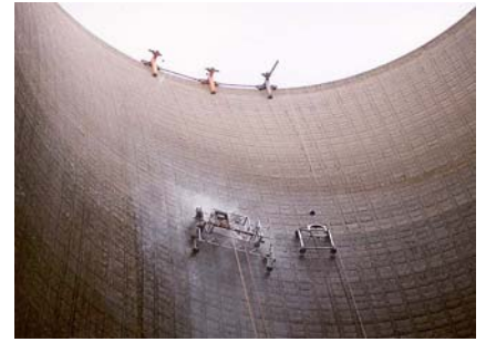
Cooling tower internal cleaning
